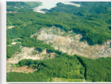
Hillside collapse that occurred in virtually all of the Hiyashizawa valley side slope
